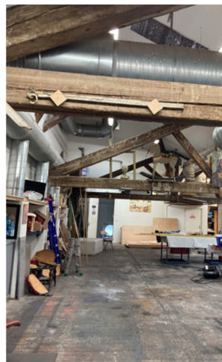
Zone D - Charpente
